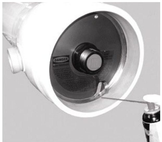
Applying penetrating fluid
